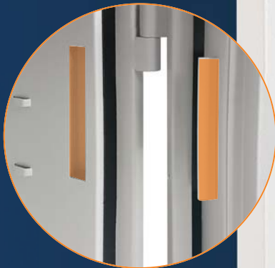
Dead bolts on hinge side
